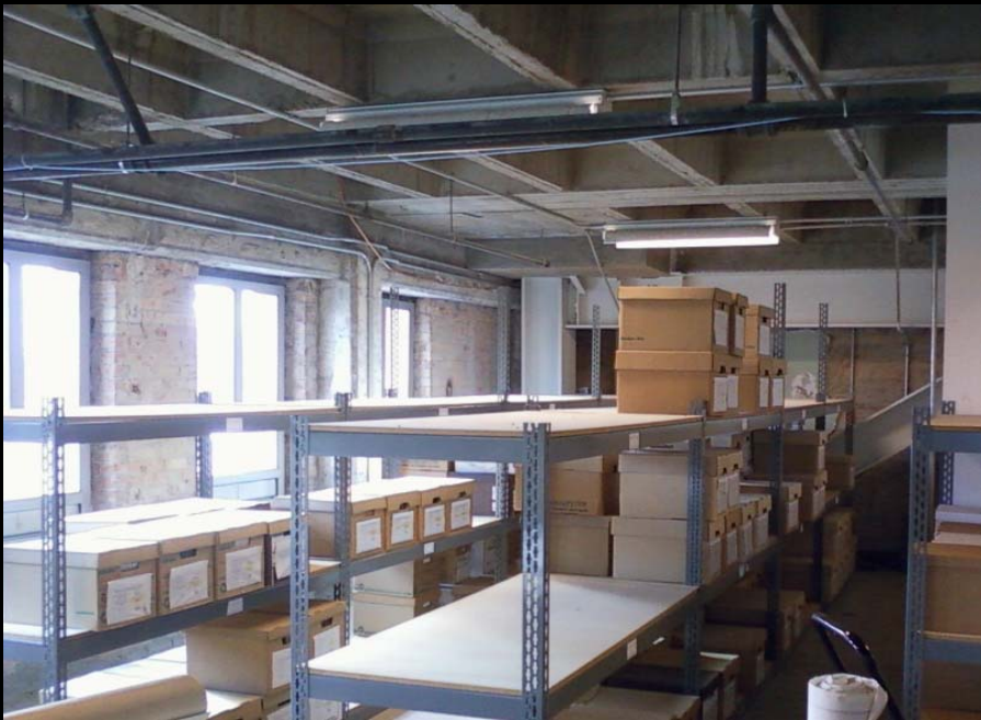
Large windows with no coverings Also known as the fly graveyard
